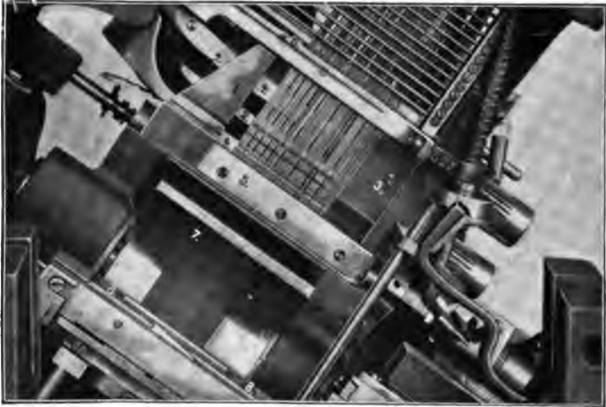
Fig. 121. Vice-jaw closed but Line not yet justified.
