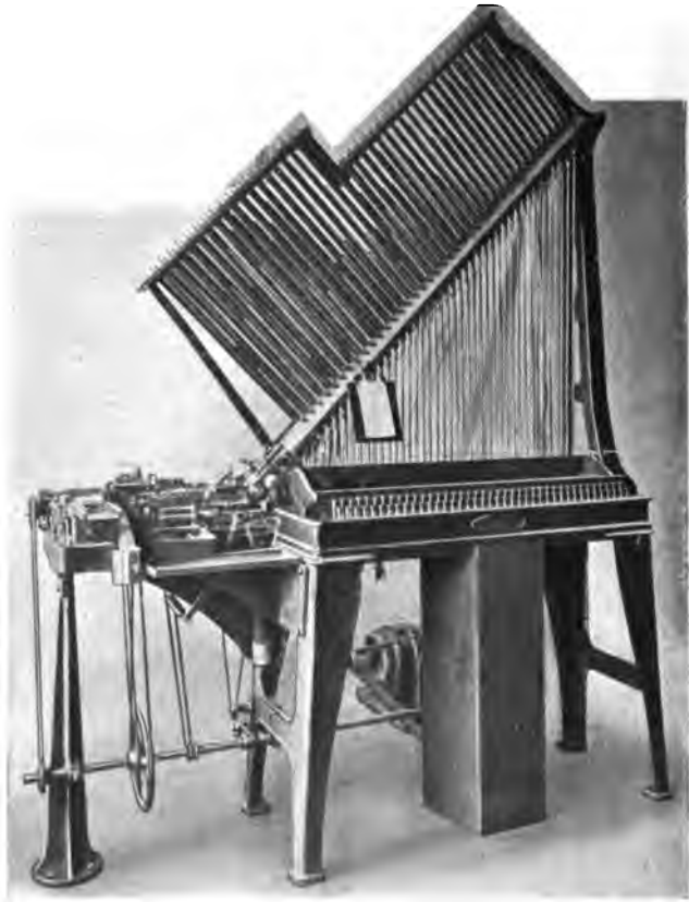
FIG. 315.— Wicks composing machine ; with Stringer line-justifier attached.
