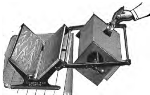
APPLYING THE CEMENT.
