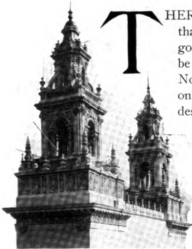
TOWERS OF MACHINERY BUILDING.
