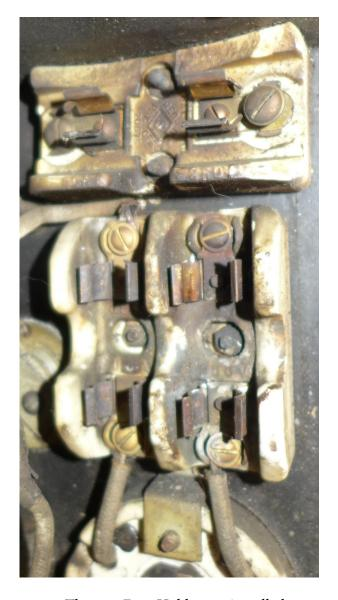
The two Fuse Holders as installed on the inside of the Right Side of the Main Electrical Enclosure
